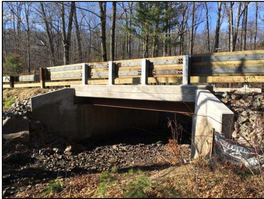
Red/Yellow Loop Trail Bridge
